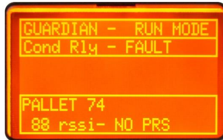
Figure 16: Condition Relay Status (No Pressure)
